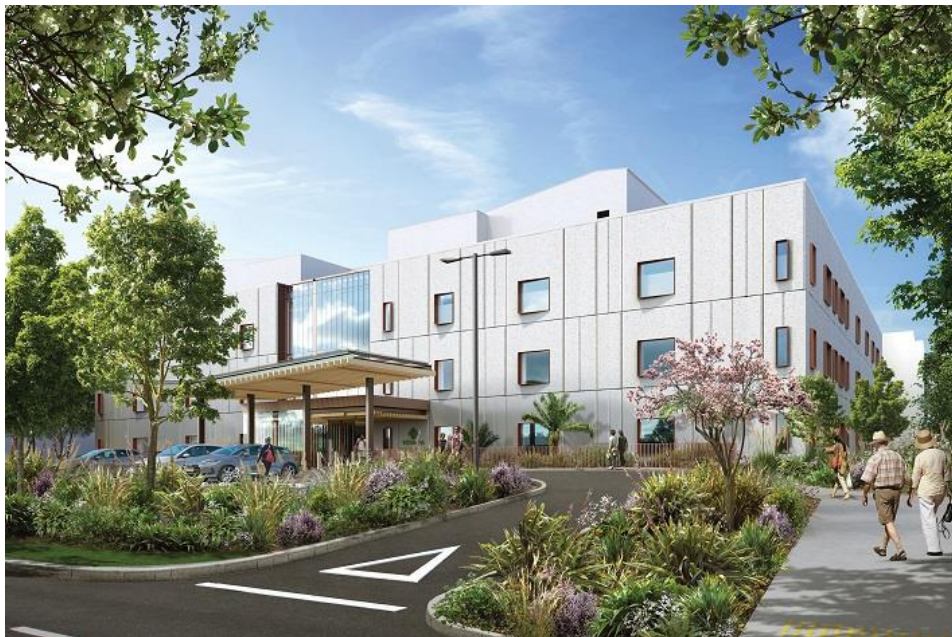
Above: an artist's impression of Tōtara Haumarū, Waitematā DHB's new hospital building, under construction at the North Shore Hospital campus.
